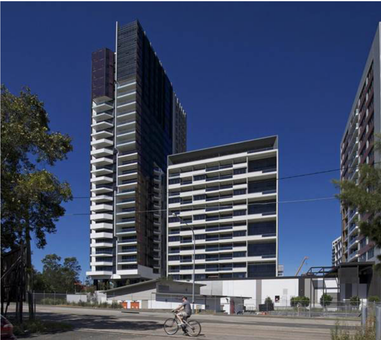
Victoria Square North: 20 Gadigal Avenue, Zetland, NSW, Australia – Floorplate: 700sqm including balcony – Floorplate dimensions: 46m x 15.2m = 700sqm. – Building Height: 85m and 26 storeys – Slenderness ratio: 1:6 (using the narrow side of the building)
